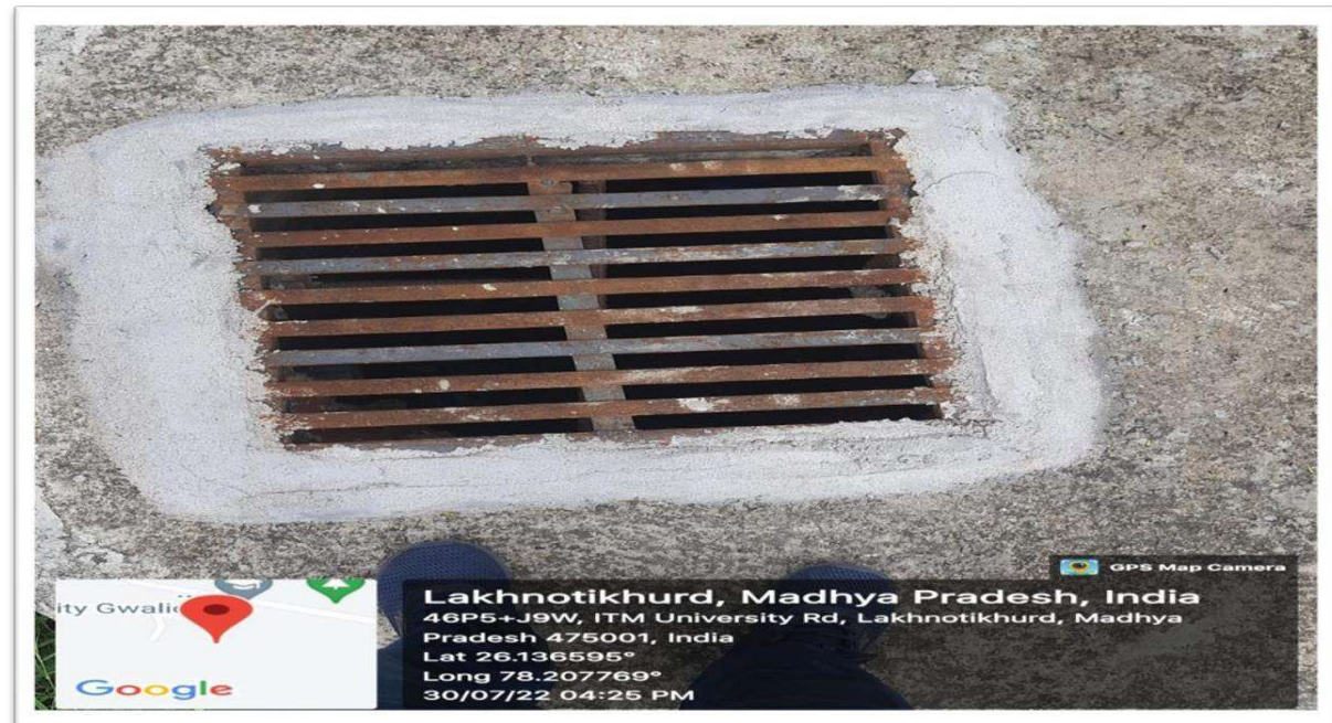
UG Tanks Near LDV Block
